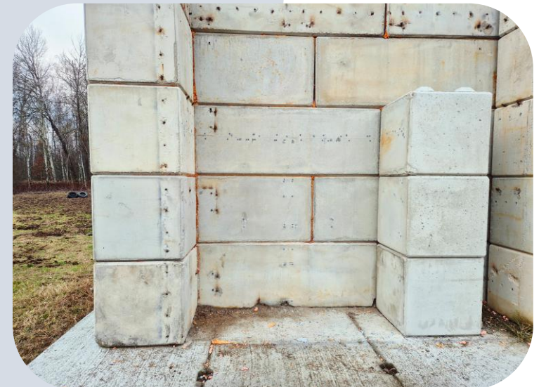
Wall after explosions
